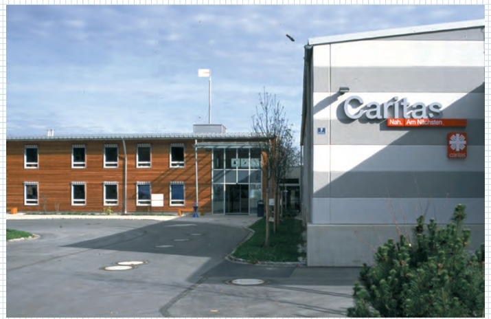
"Charity shops" in Obermühl (Raubling) heat with the HDG Compact 200
