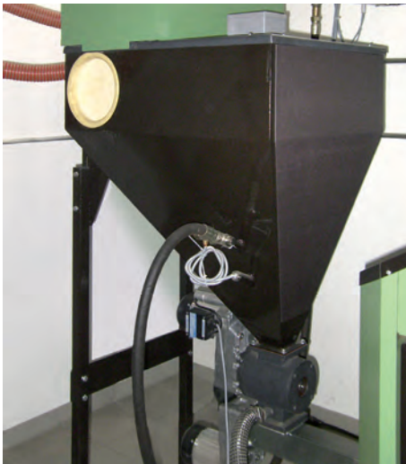
The intermediate container of the HDG pellet suction system can hold up to 100 kg of pellets.
