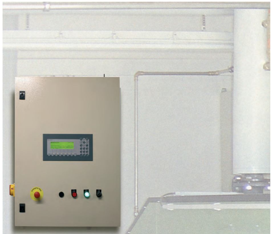
All components of the system are electronically controlled by a PLC controller inside the control cabinet. Current operating data from the combustion system is indicated on an illuminated display.
